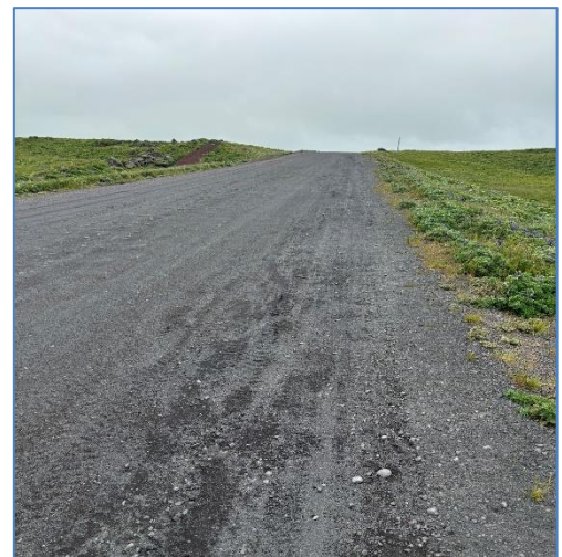
Areas of road to airport need improvements
